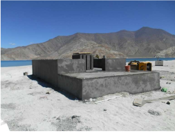
Figure 4.4: The telescope pier and the walls constructed for installation of the H-alpha telescope at Merak.
