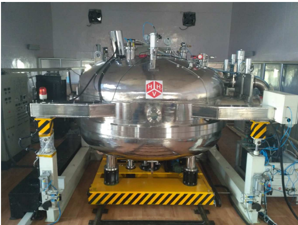
Figure 4.3: Fully installed coating plant.
