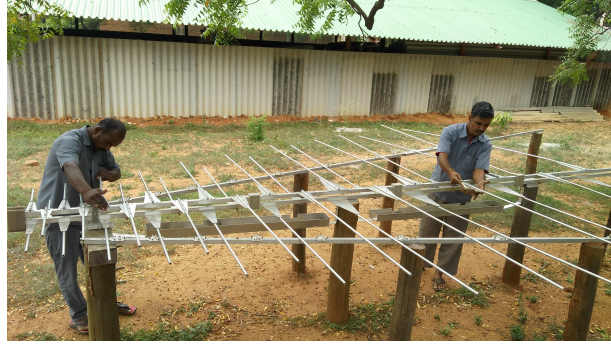
Figure 4.17: Assembling of the LPDA in the Gauribidanur observatory.
