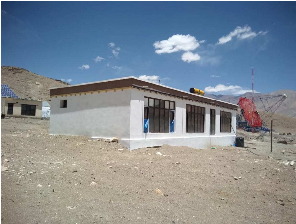
Figure 4.7: Staff accommodation at IAO, Hanle.
